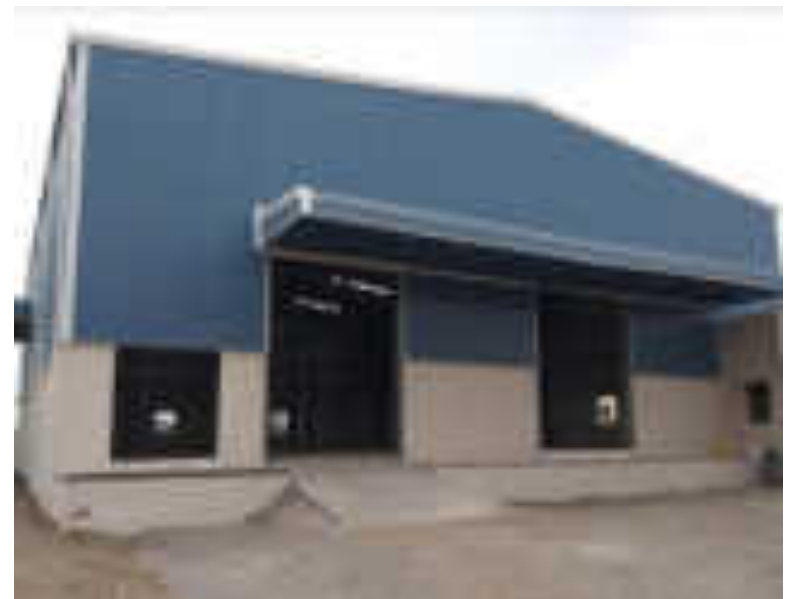
PEB construction works
