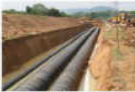
MS PIPE LAYING WORKS - PRELIMINARY STAGE
