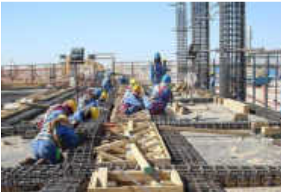
Civil structural Works
