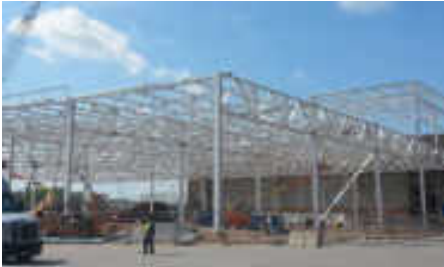
Mechanical Structural Works
