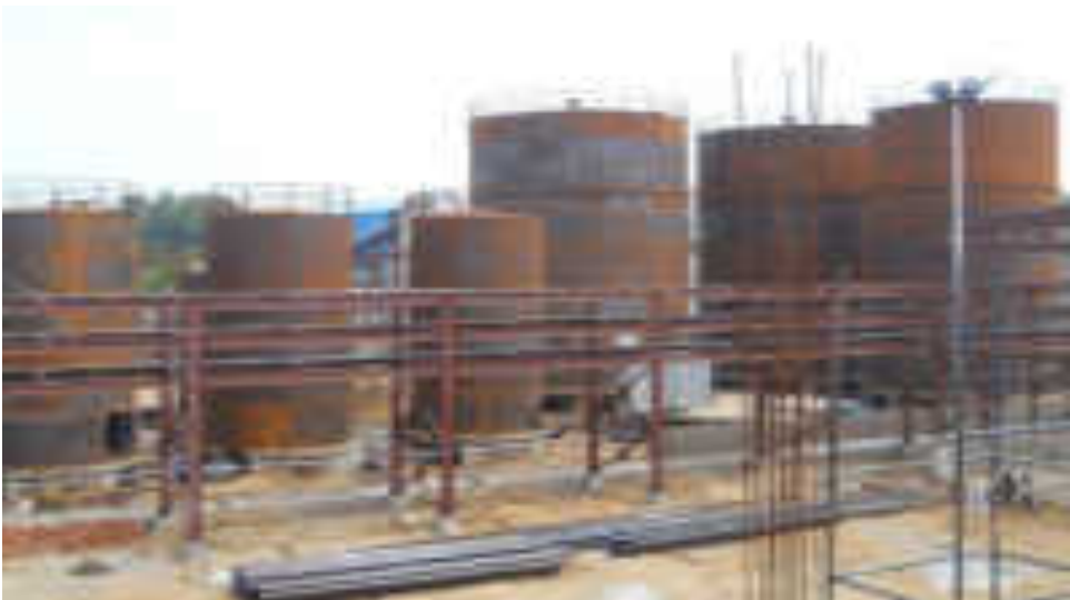
Process and Maintenance tank formation
