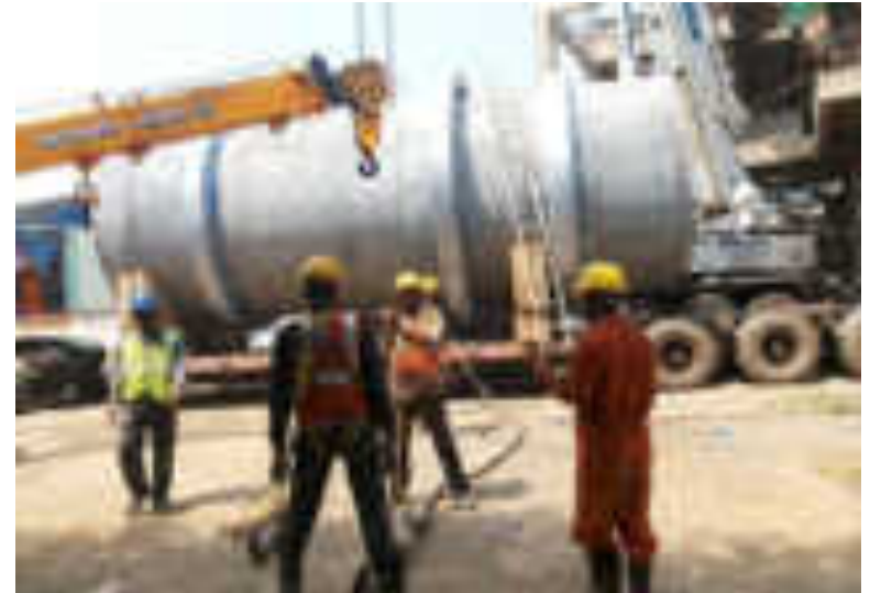
Equipment Erection works
