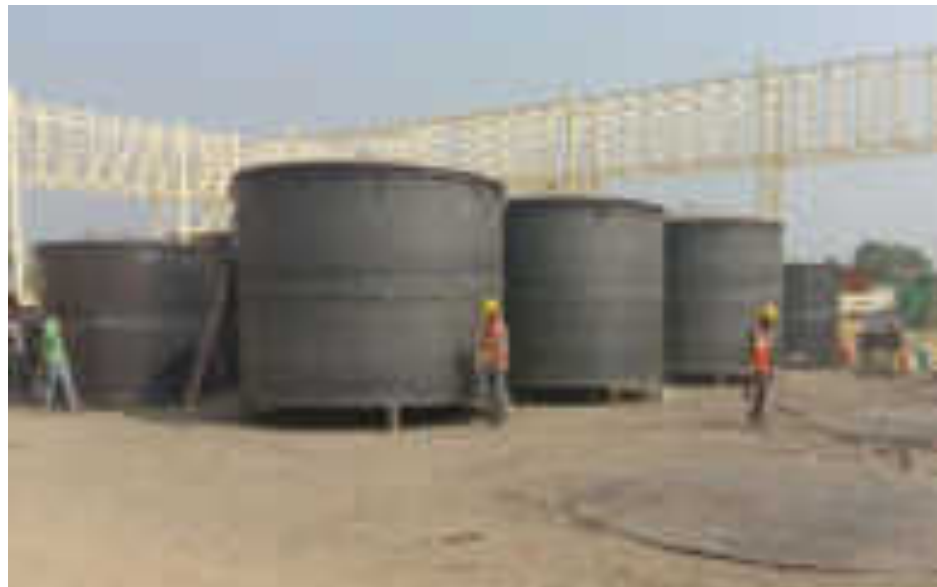
Tank and pipe erection
