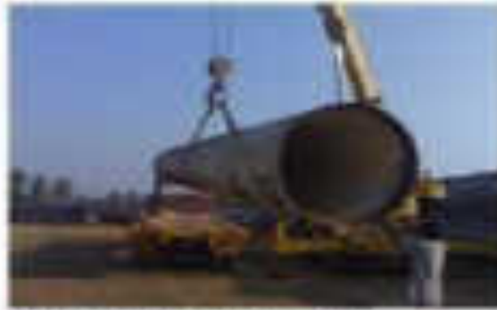
MS PIPE LIFTING WORKS - HEAVY LIFTING PLANT
