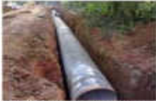
MS PIPE LAYING WORKS - PRELIMINARY STAGE
